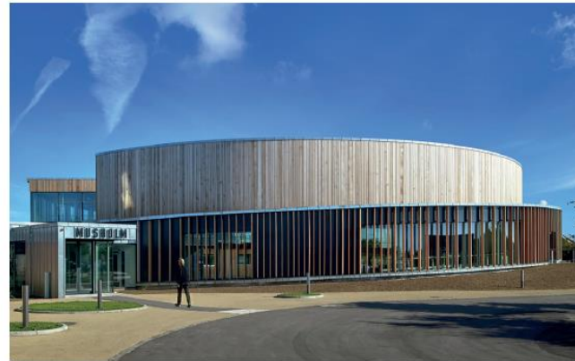
Musholm Extension, Denmark
