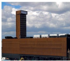
Olympics energy centre, Stratford
