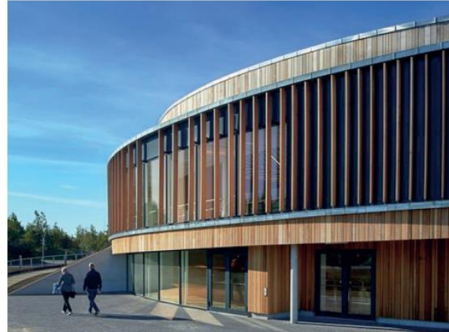
Musholm Extension, Denmark
